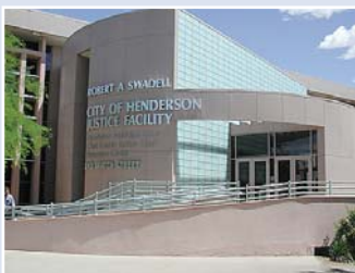
Robert A. Swadell Justice Facility. To fund part of the project costs for the Justice Facility, savings were used from retrofitting traffic signals at over 64 intersections to LEDs.
